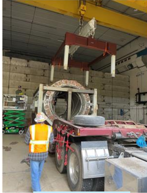
IR12 Calorimeter removal
