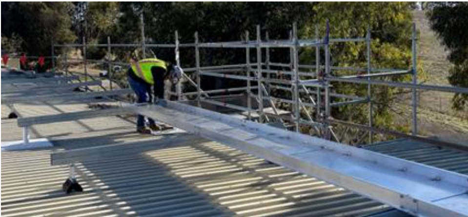
Installation of roof-mounted cable trays. Mockup completed and actual installation in progress
