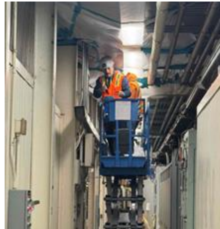
Installation of roof-mounted cable trays. Mockup completed and actual installation in progress
