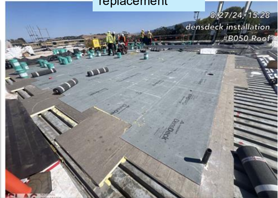
B050 Roof replacement
