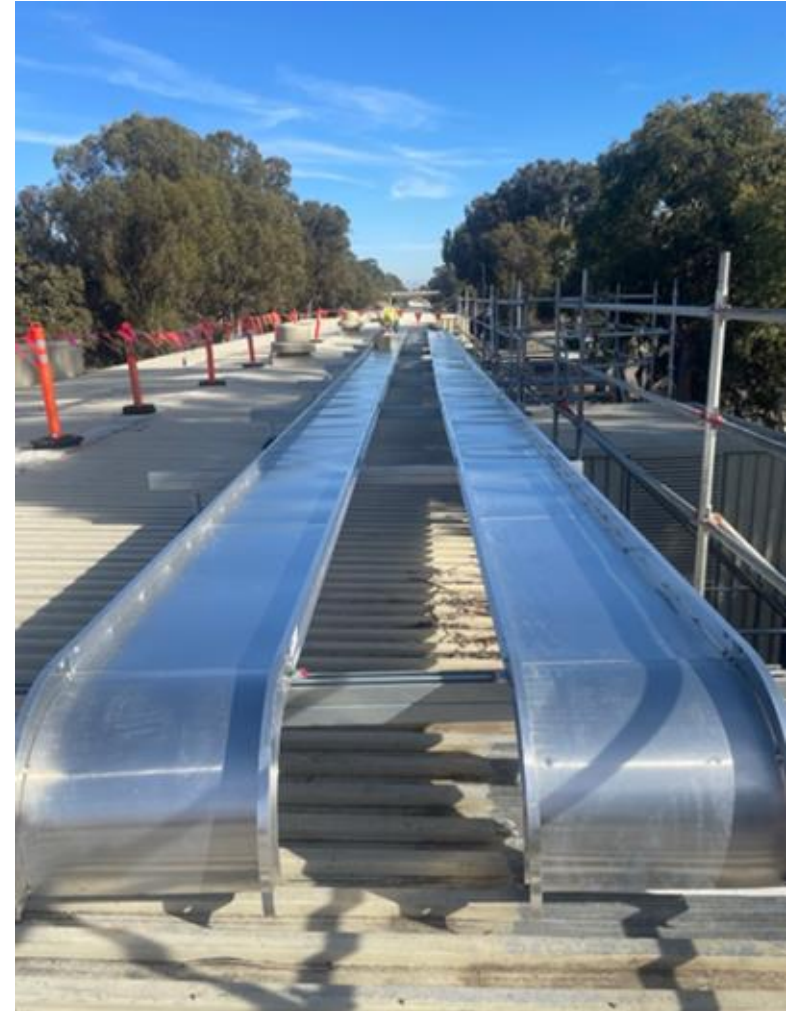
Installation of roof-mounted cable trays. Mockup completed and actual installation in progress
