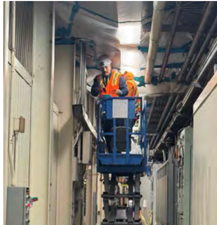
Installation of roof mounted cable tray mock ups
