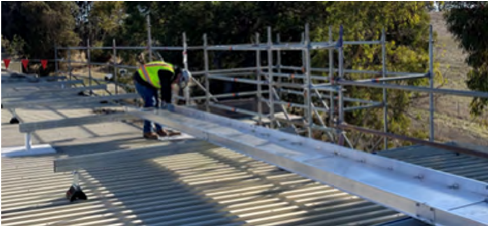
Installation of roof mounted cable tray mock ups
