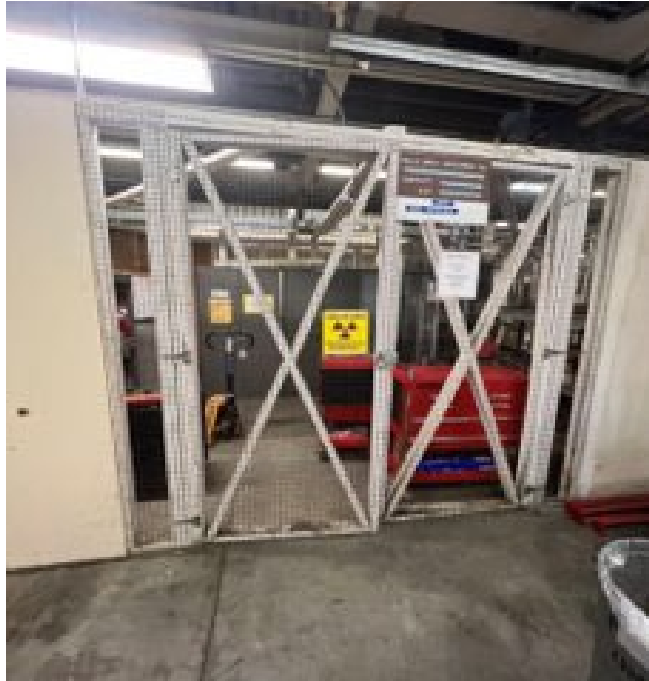
Radioactive material (RAM) stored in Sectors 11 to 30
