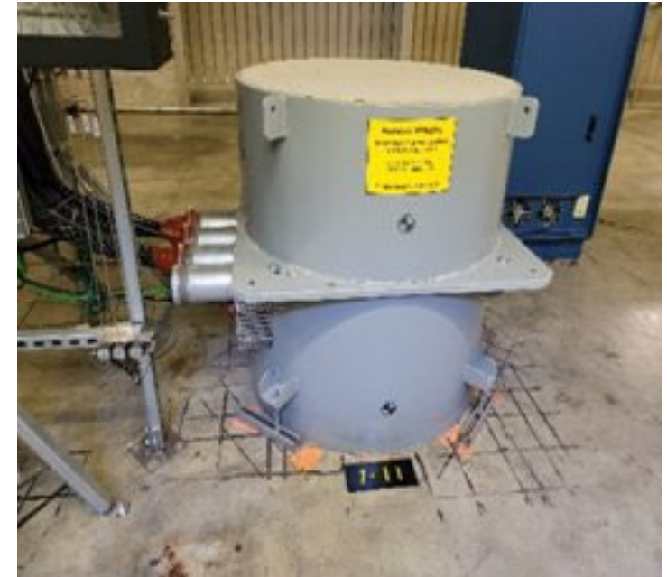
Penetration Shielding Shielding for penetrations Sectors 0 to 10
