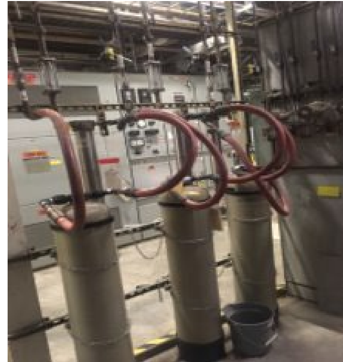
17 potentially radioactive Low Conductivity Water (LCW) Systems in the gallery. Example: Sector 30 Magnet Resin Bottles
