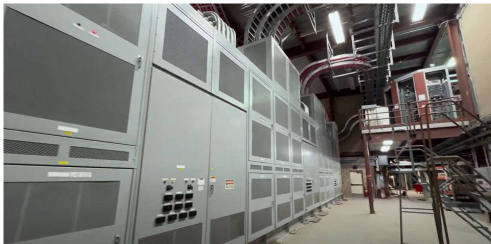
Internal view of MSS B016
