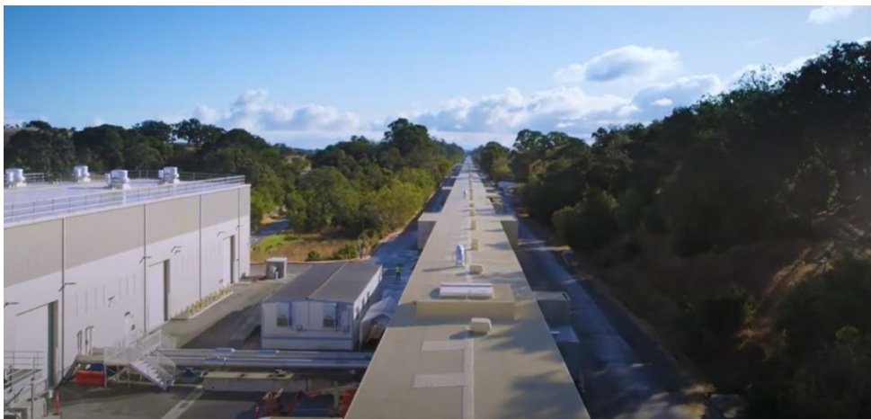
Existing Klystron Gallery Roof
