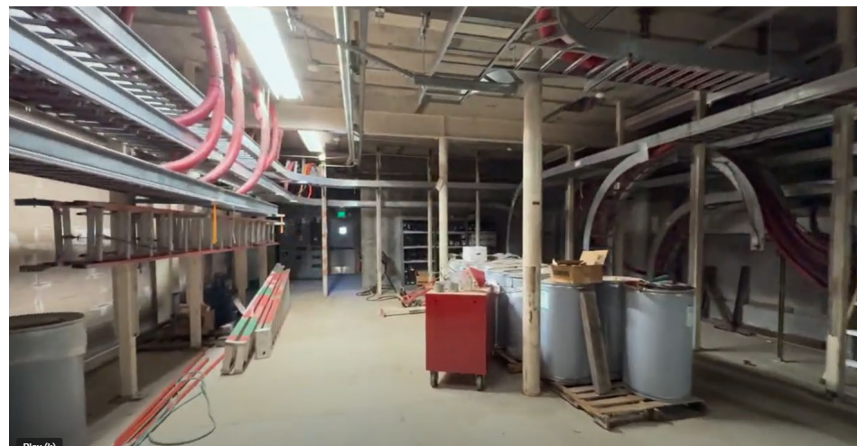
Internal view of MSS B016
